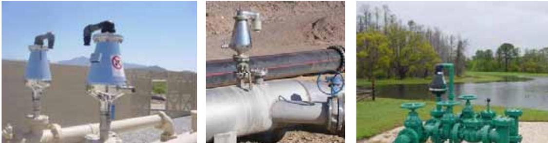
Figure 13: Stainless steel and composite material combination air valve for wastewater
